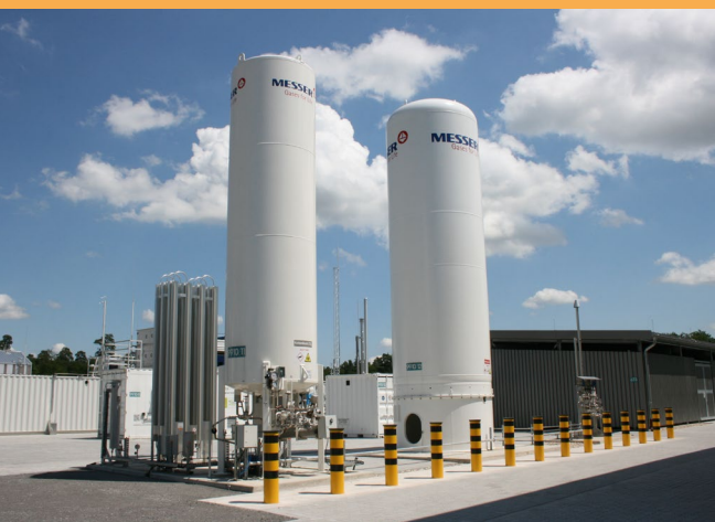
Hydrogen tanks at KIT. Photo: KIT
