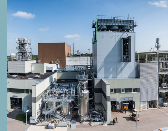
The pilot plant demonstrates all stages of the bioliq® process: Flash pyrolysis, high-pressure entrained-flow gasification, hot gas cleaning, and synthesis. Photo: KIT
